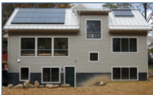
Left: The rear roof of the house, which faces south, is equipped with a 3.12 kilo Watt PV system and evacuated tube solar hot water. Right: North face with few windows.
